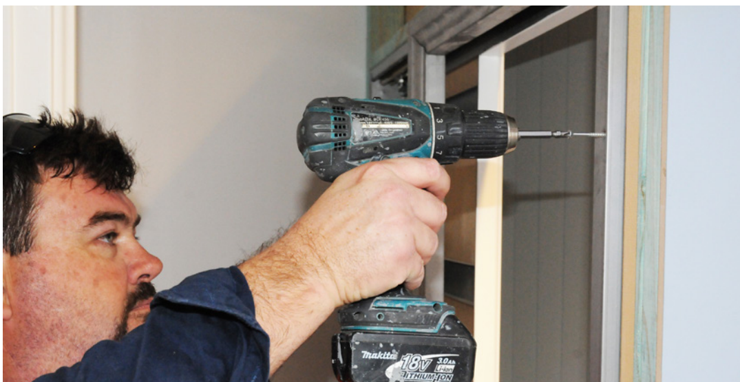
Architrave fixing through counter sunk
